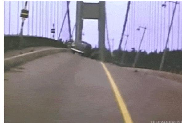
Tacoma Narrows Bridge oscillating and collapsing because oscillatory winds blew at its resonance frequency. (collapsed under 64 km/h wind conditions the morning of November 7, 1940)
